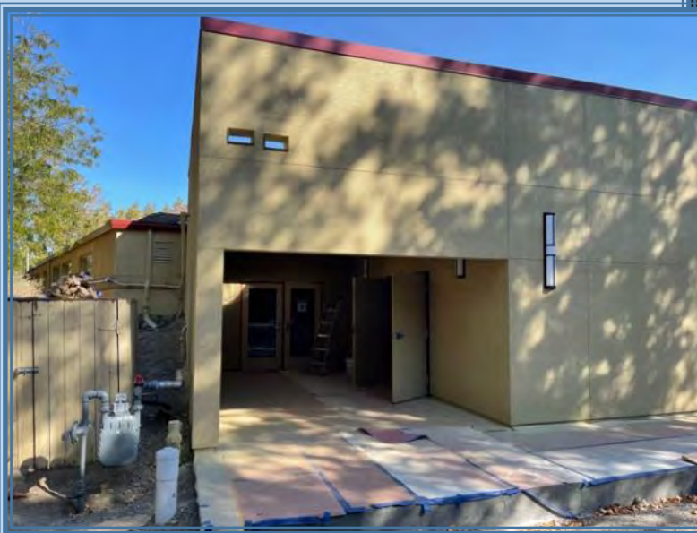
Exterior paint, including the trim is complete.
